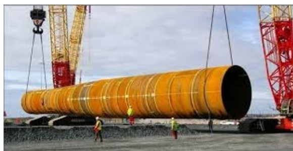
Figure 15 Horizontal monopile lifting (2 points)
