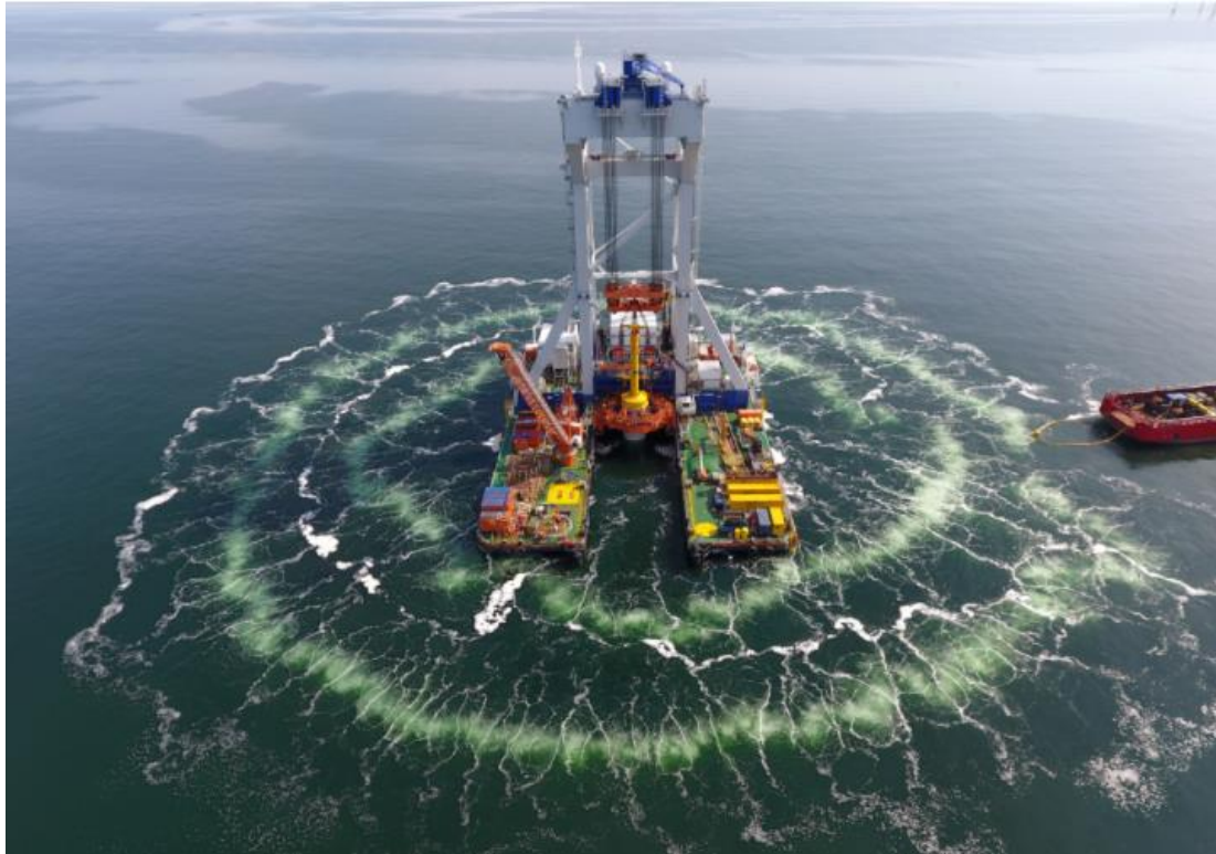
Figure 4-1: Van Oord's Heavy lift vessel Svanen [source ("Vesselfinder.com," 2020)]
